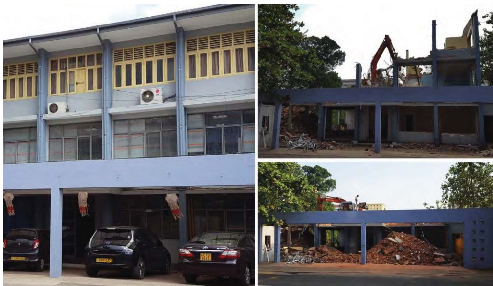
Figure 77: Old building of NSACP demolished in 2016
