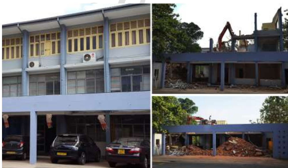
Figure 76: Old building of NSACP demolished in 2016
